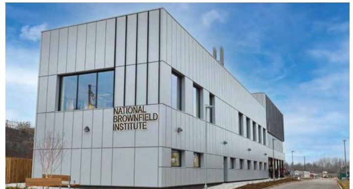
The new National Brownfield Institute (NBI) in Wolverhampton, part of the University's Springfield Campus focusing on brownfield development including contaminated land.
