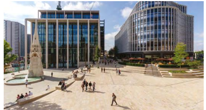
The £700 million Paradise development in Birmingham is one of the largest and most strategically important city centre schemes outside of London.
