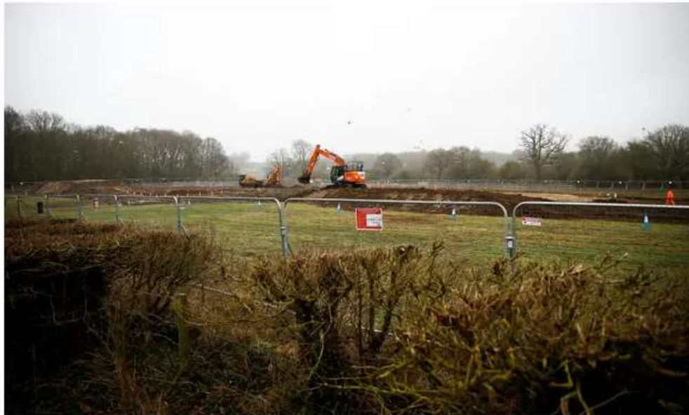
▲ Work under way along the route of HS2 in Harefield, north-west of London, in January 2020. Photograph: Henry Nicholls/Reuters
