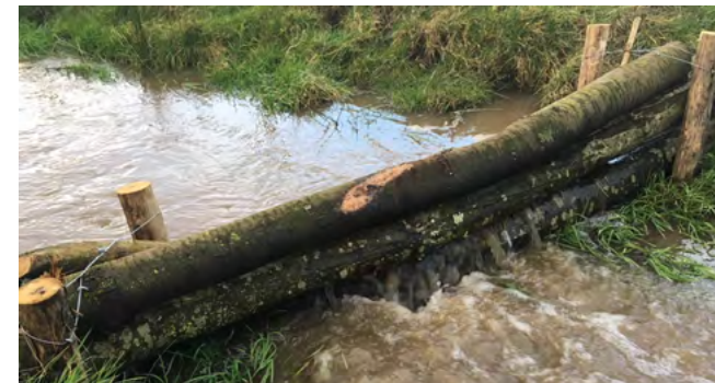
Figure 3-1: “Leaky barriers” help to reduce flow and capture pollutants, and are simple nature-based solutions (© The Wildlife Trusts)
