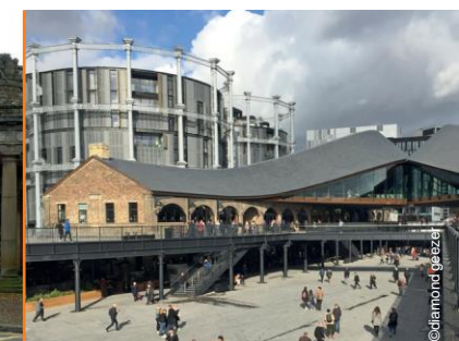
Coal Drops Yard, London Industrial to retail
