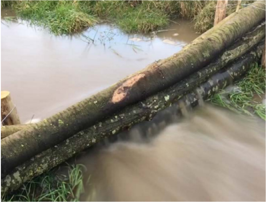
Figure 3-1: “Leaky barriers” help to reduce flow and capture pollutants, and are simple nature-based solutions ( © The Wildlife Trusts)
